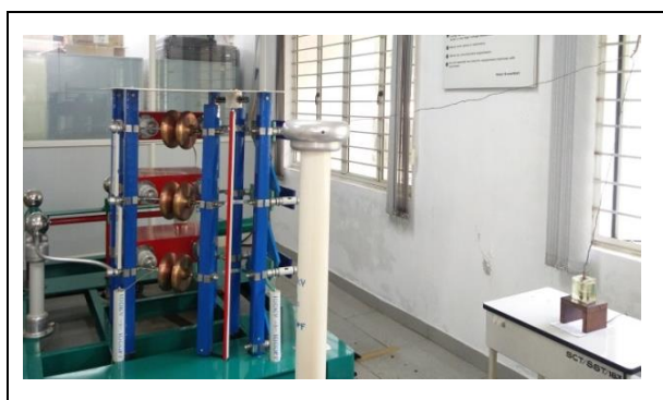
Fig. 2: 3-stage, 300 kV Lightning Impulse Generator connected to the test cell.
