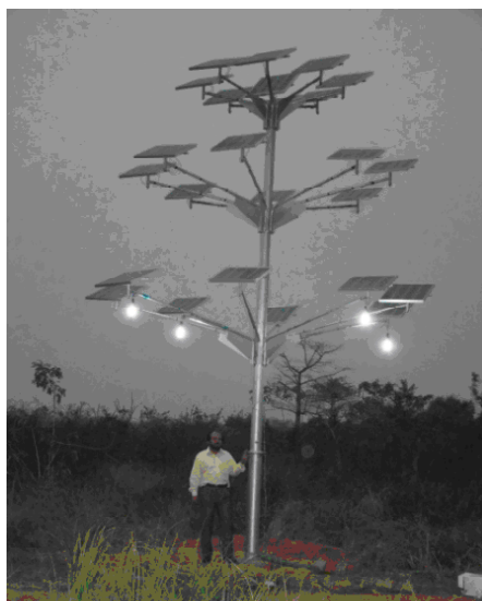
Fig. 9b: Solar Power Tree At Night
