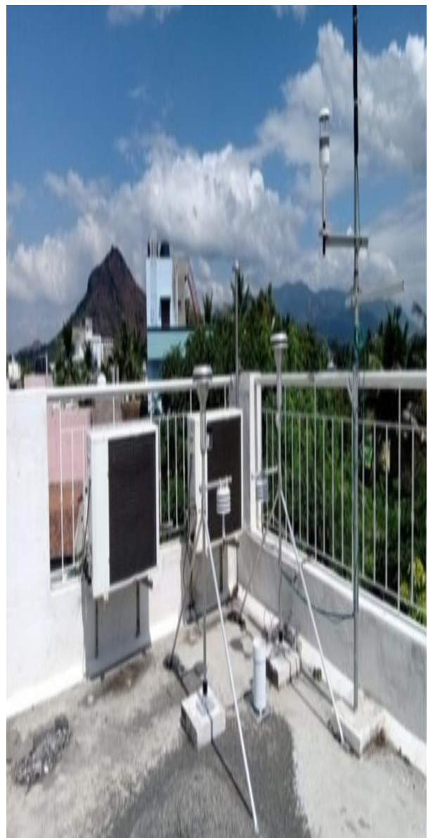
Fig. 3: Air Quality Monitoring System
