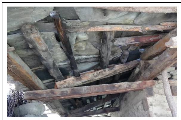
Fig. 6: Wooden rafters & purlins.
