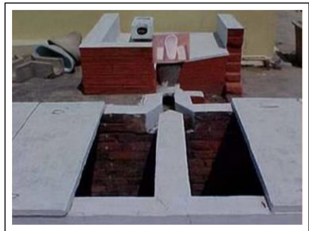
Fig. 6: Two pit sanitation system
