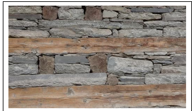
Fig. 3: Timber tie bands.
