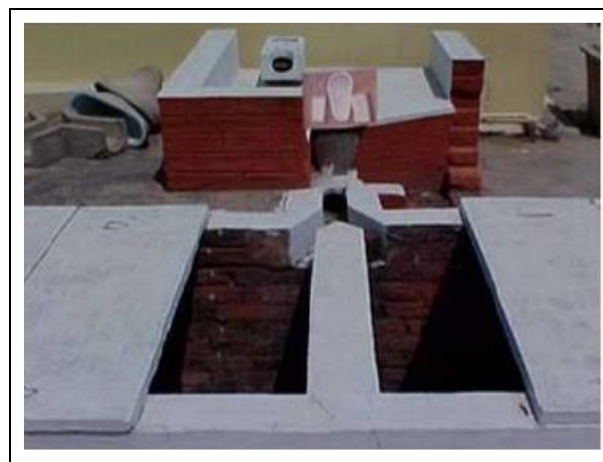
Fig. 6: Two pit sanitation system
