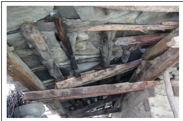
Fig. 6: Wooden rafters & purlins.
