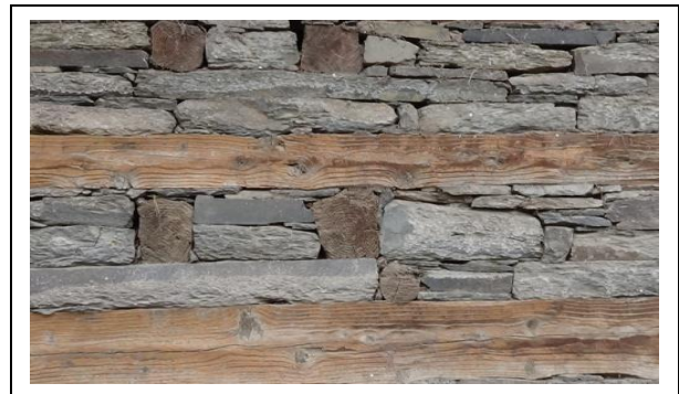
Fig. 3: Timber tie bands.
