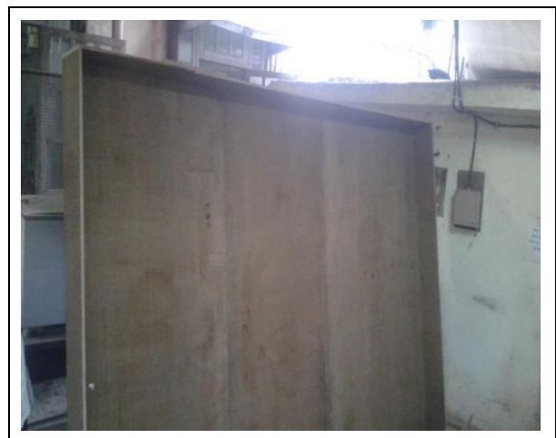
Fig. 8: Mould forcasting of wall/ slab panels.
