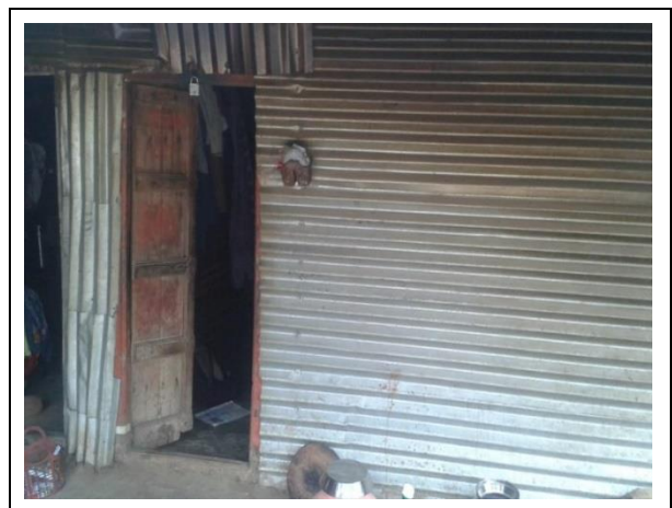
Fig. 5: House using metal sheets.
