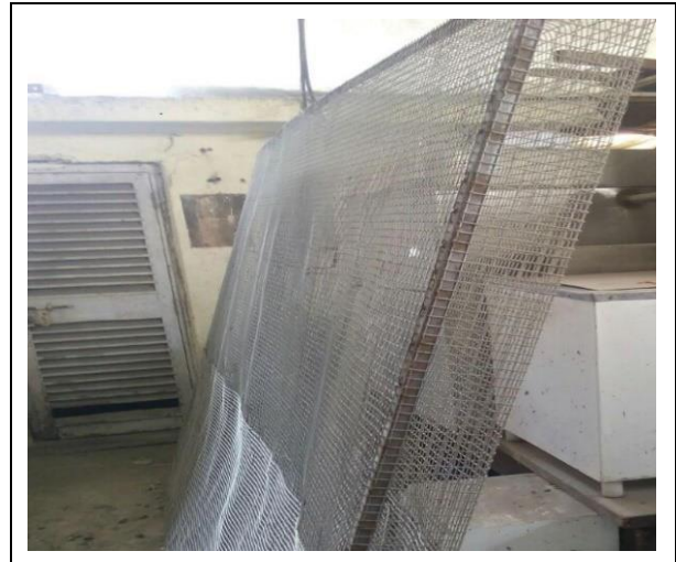
Fig. 7: Wire mesh for wall / slab panels.
