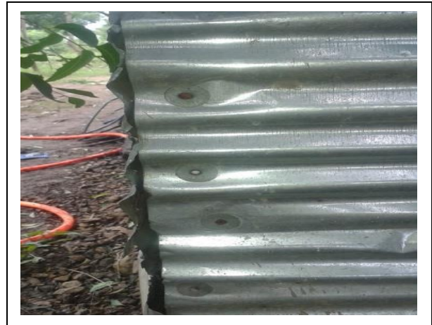
Fig. 6: Connection details of metal sheet house.
