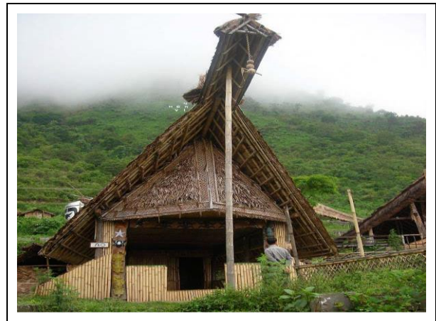
Fig. 5: High pitched roof Kutchha House [24].
