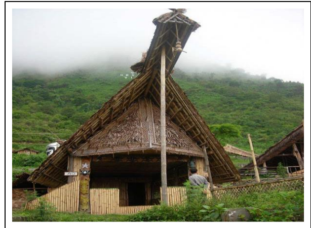
Fig. 5: High pitched roof Kutchha House [24].
