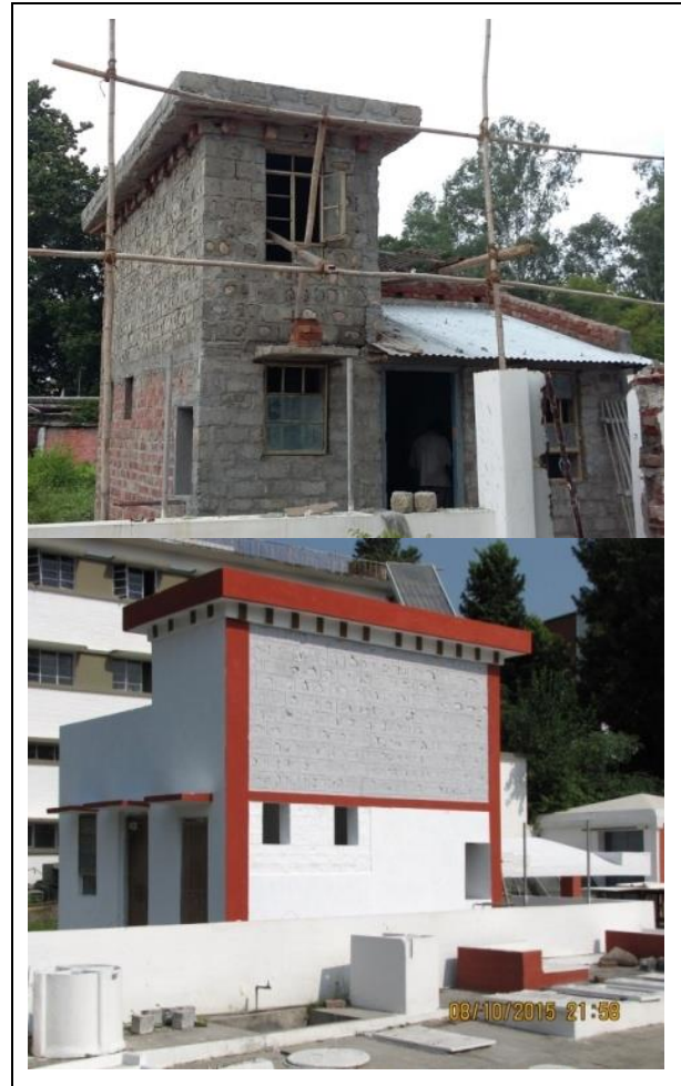
Fig. 3: Construction of the prototype in Rural Park at CBRI, Roorkee.
