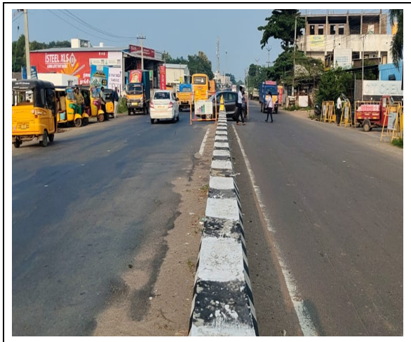
Fig. 9: Location for laying paver block footpath
