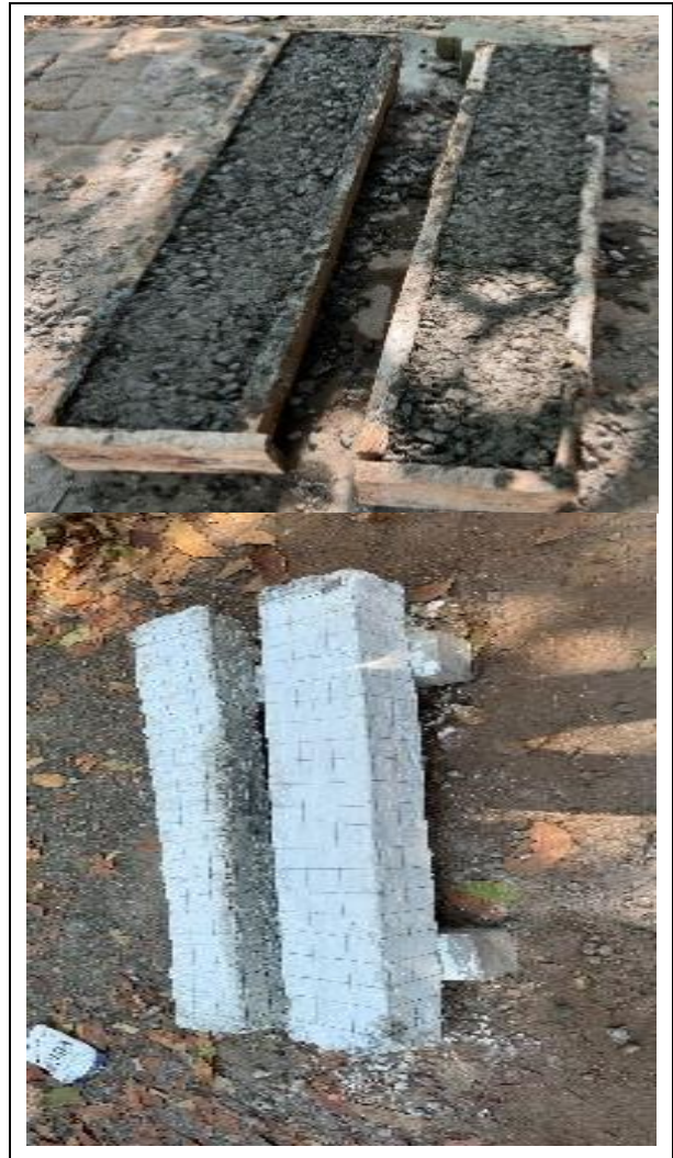
Fig. 7: Casting of beams
